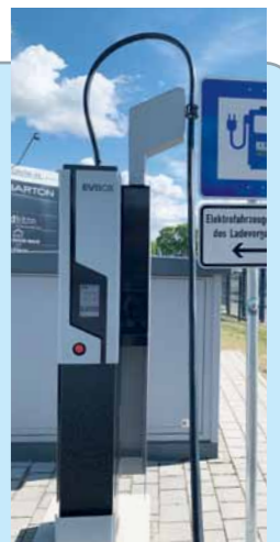
Peculiar: At this station, the charging cable is clamped between the information signs.
